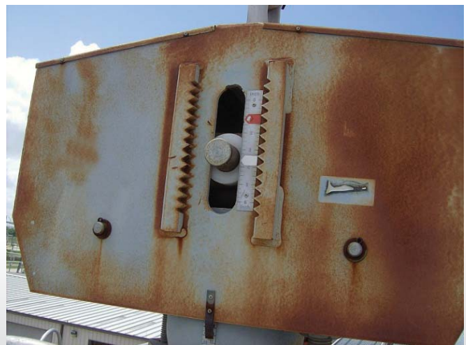
Figure 10 - Real World Example of Paint and Lack of Cathodic Protection
