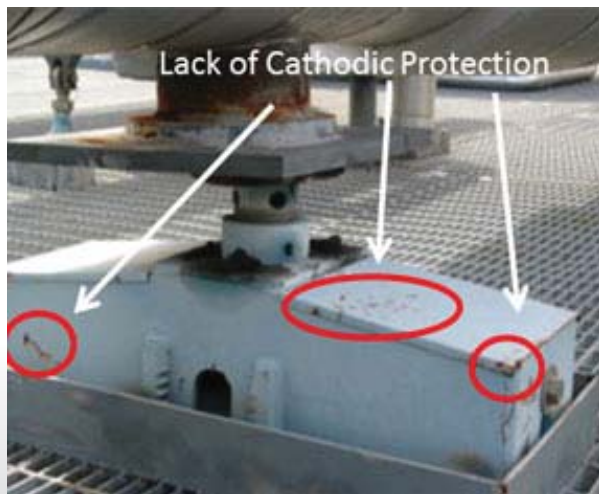
Figure 10 - Real World Example of Paint and Lack of Cathodic Protection
